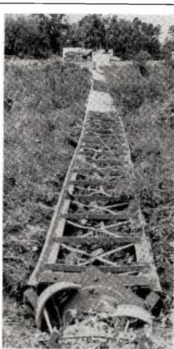
Tornado topples tower
